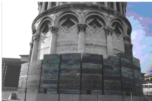
Figure 7. Lead counterweight on the North Side.
